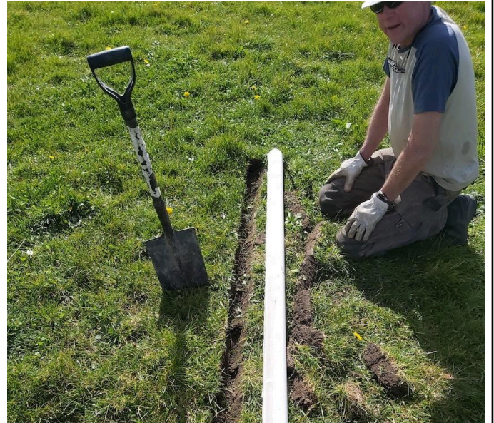
Step 7: Dig trench for collector
