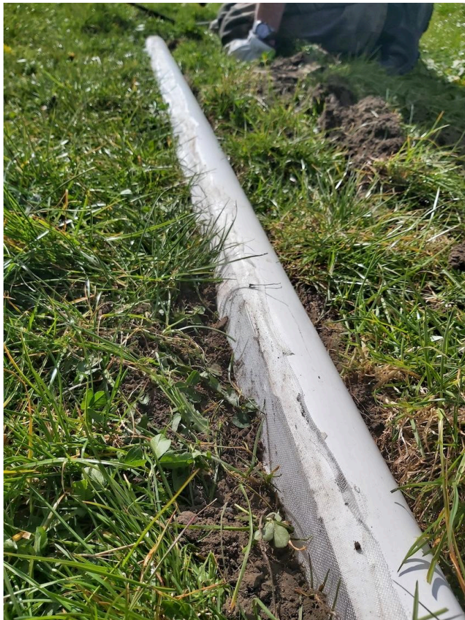
Steps 10-12: Fill the trench with slurry and install collector with mesh slightly below soil surface
